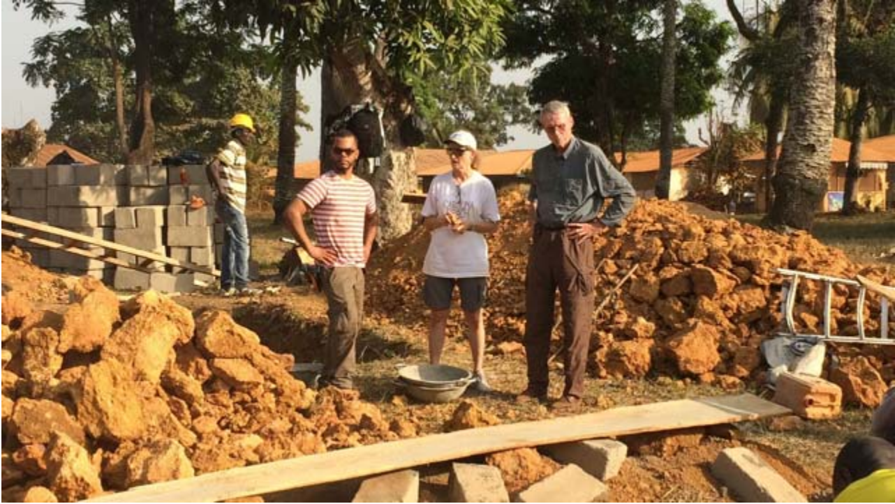
Jose, Joan and Tom at the construction site
