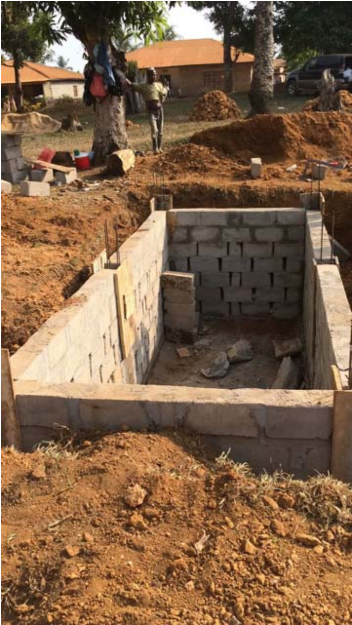
The Cesspit walls are also up
